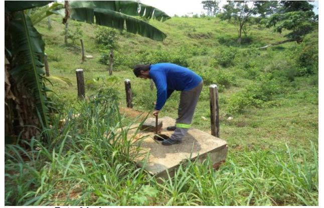
Foto 04: descarga; S 10°15'30.6'' W063°45'15.8''
